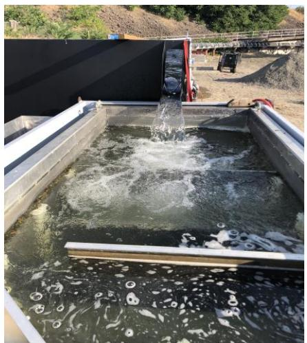
Pictured here are the collection tank and the discharge point on the downstream end of the dewatering screen.
